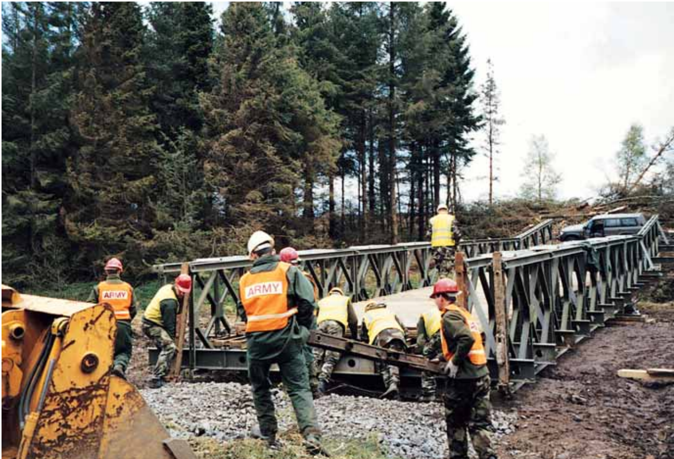
Construction of a Bailey Bridge.
